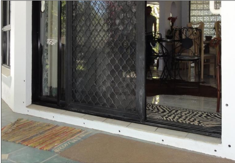
Figure 8: Drill holes around a resident's external doorway ready to install a sheet of marine plywood to help prevent water from entering the home
